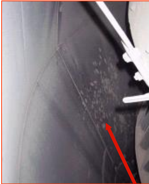
Liner plates on walls Erosive wear HARDOX 400, 450
